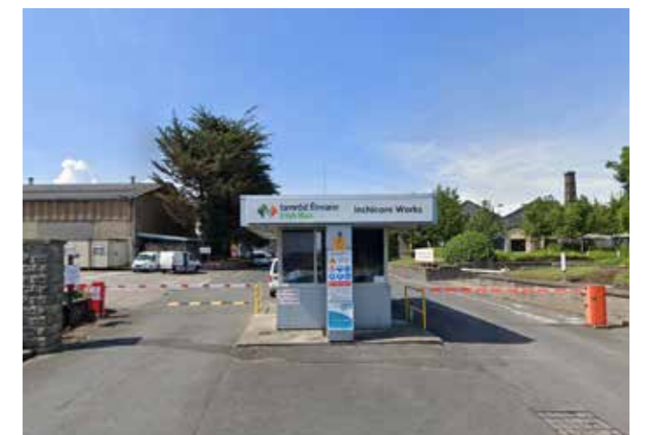
Irish Rail Works Site
